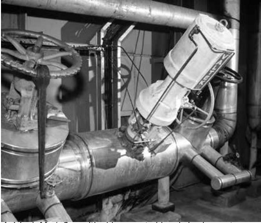
A 4-inch Mark One with side-mounted handwheel operates a boiler feedwater system at a pulp plant.
