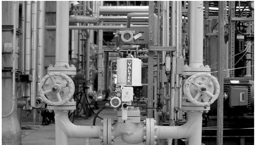
This 8-inch back-pressure control valve operates in a liquid hydrocarbon plant with a 580 psi/40 bar upstream pressure
