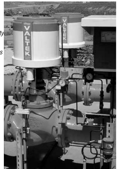
(Left) Mark One valves used to operate a PSA skid.
